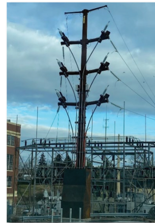
Wire and Terminations complete on the Riser pole near Hershey Substation
