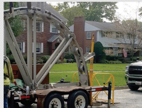
Underground Cable pulling rig set up on Elm Avenue
