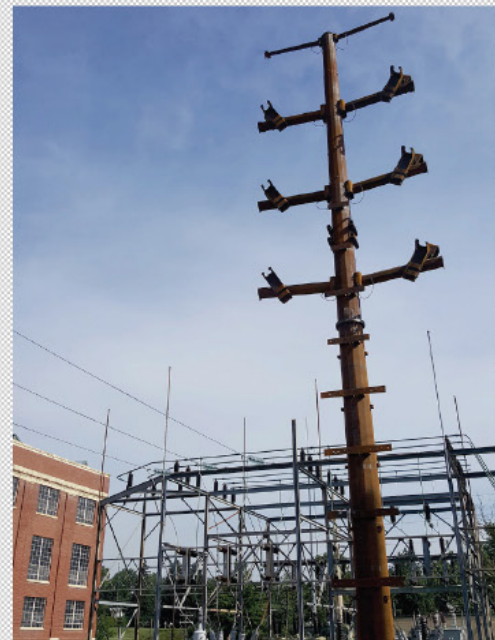
Hershey Substation Riser Pole near Old Hershey Chocolate Factory
