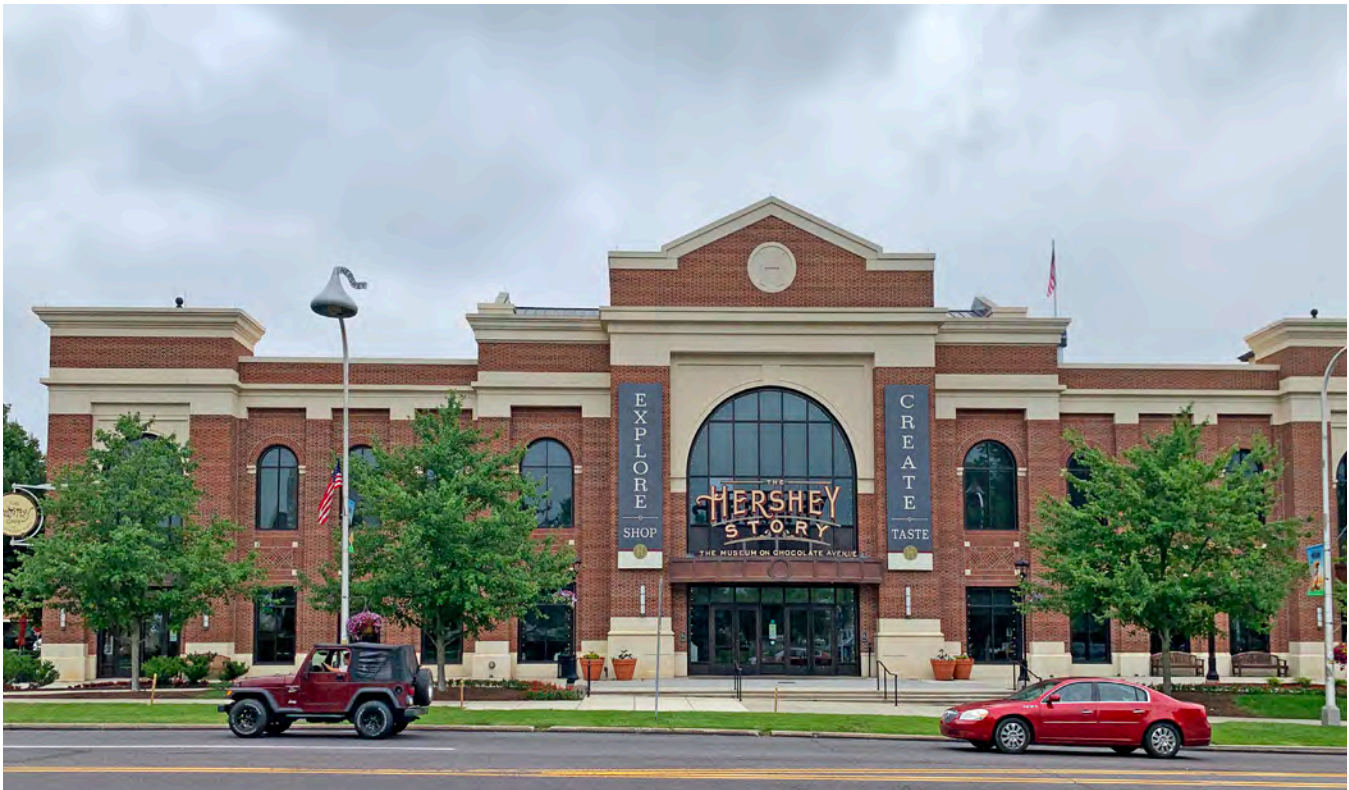
Figure 17.8 An example of new construction that uses materials contextual to the region and in a way reminiscent of Hershey's industrial past.
