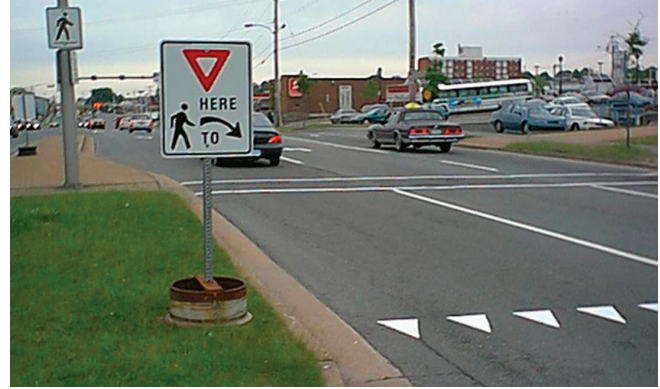
Advanced yield markings are recommended in conjunction with uncontrolled pedestrian crossings on multi-lane roadways to reduce the possibility of multiple threat crashes.
