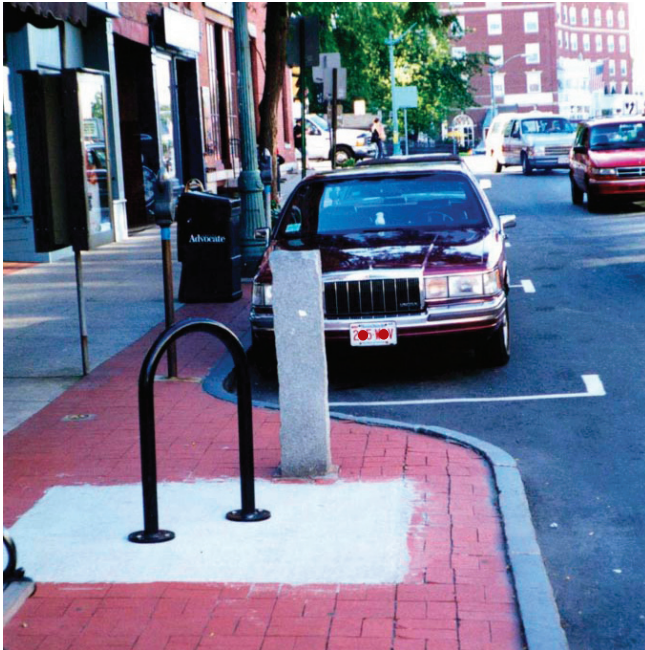
In addition to improving sight distance of and by pedestrians, a curb extension provides room for a bike rack in a constrained urban area.
