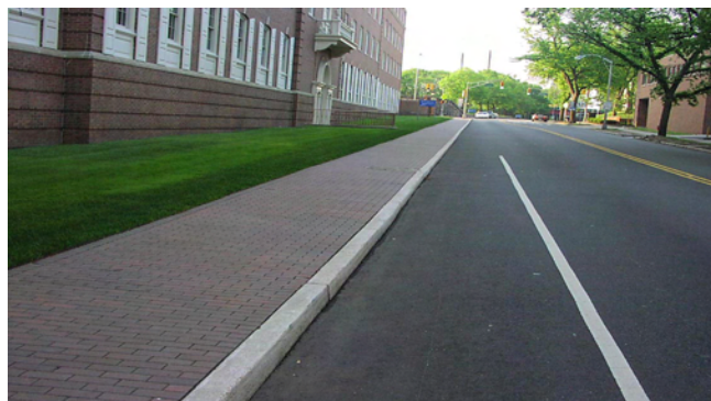
Rutgers University in New Brunswick, NJ striped a shoulder on George Street through its central campus as the most expedient way to create a facility for bicyclists.
