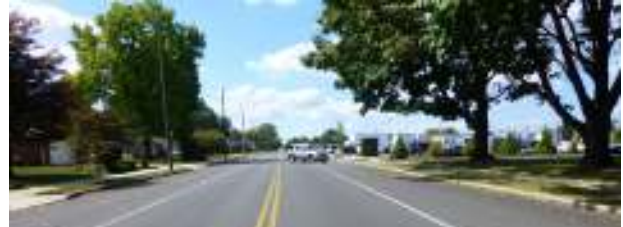
Several roadways have excessive capacity, such as Cherry Street in Palmyra (10 ft travel lanes & 14 ft on-street parking) where there is ample room to accommodate a bicycle lane and maintain parking. Additionally, there is a concrete barrier dissecting the street that was likely installed to mitigate through-traffic. Installing a bike-ped cut-through will improve access to the street for bicyclists while still prohibiting vehicles.
