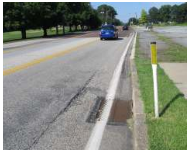
Stormwater grates are a hazard for people on bicycles. Many are placed in spaces where bicyclists are expected to ride, forcing riders to maneuver into the travel lane to avoid them. Many grates in the study are placed incorrectly for bicyclists, causing bicycle tires to get caught and injuring riders.
