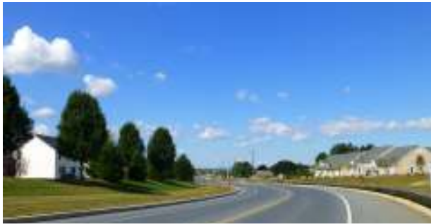
Northside Drive in South Londonderry Township is an example of a curvilinear street that is common throughout the study area. The design of the road fosters high speed traffic. The width can become an opportunity to add bicycle facilities while maintaining vehicular efficiency.
