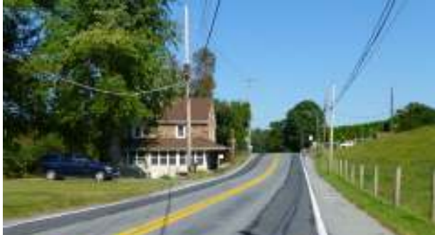
Route 241 has been identified as a Regional Bike Route by Lebanon County and is an example of a narrow roadway corridor that is constrained by utility lines. This can result in insufficient width for drivers to safely pass bicyclists.
