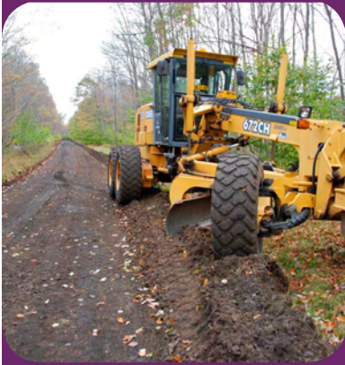
Trail Construction Black Diamond Trail Luzerne County
