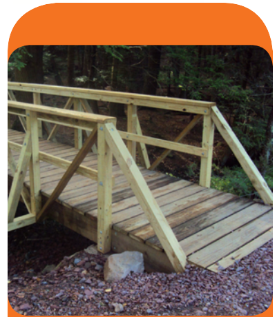
Stringer Bridge Nescopeck State Park Luzerne County
