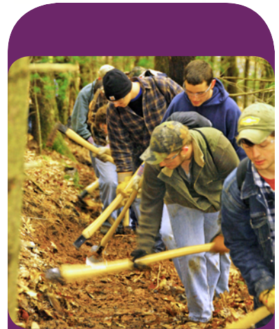
Tread Construction by Hand
