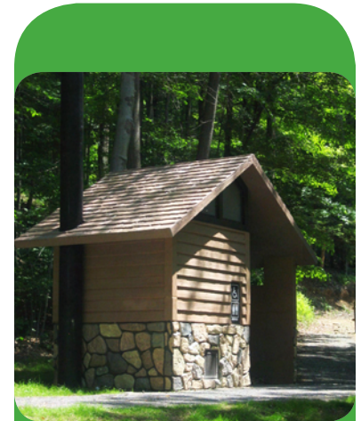
Sweet Smelling Restroom Technology Lyman Run State Park
