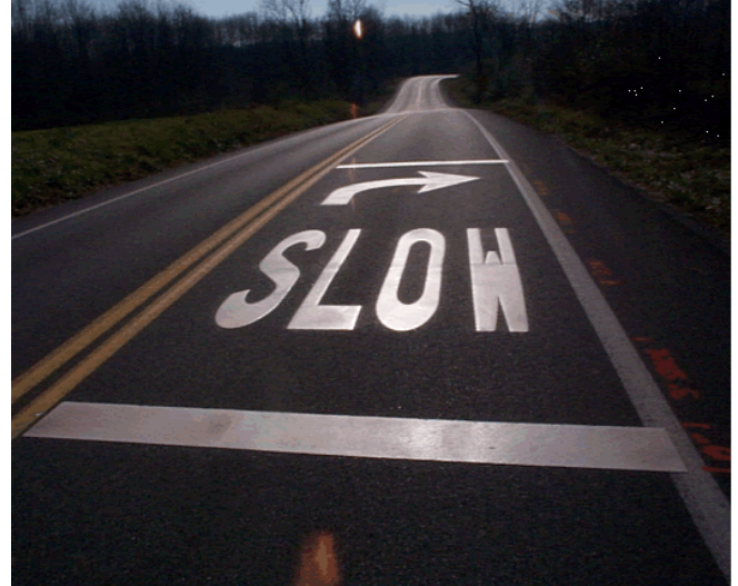
Advanced Curve-Warning Treatment
