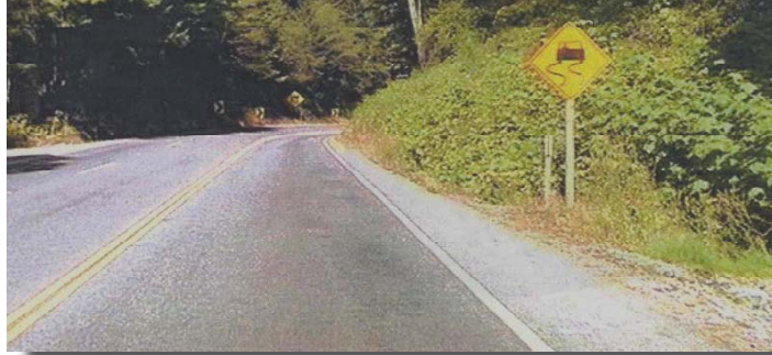
Rural curve treated with skid-resistive graded asphalt concrete, warning signs, and chevrons.
