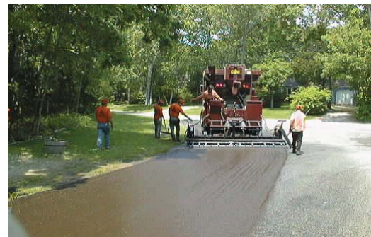
Application of skid-resistant pavement surface in curve.
