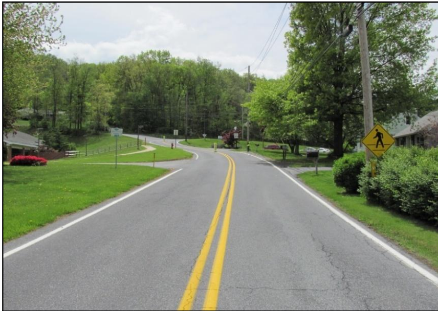
Westbound Hilltop Road Approaching Curve 2
