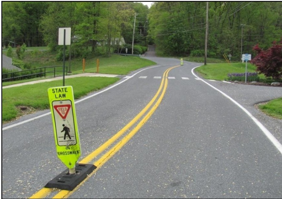
Westbound Hilltop Road Approaching Curve 1
