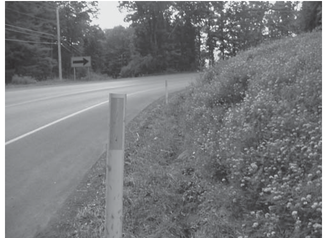
Turn delineated with reflective strips on flexible posts, Large Single Arrow sign (W1-6), and Chevron Alignment signs (W1-8) (barely visible). Note divergence of utility lines, which, in the absence of the signs and delineators, could mislead drivers about roadway alignment at night.
