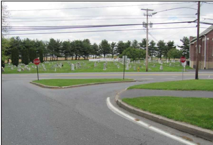
Eastbound Channelized Right-Turn Lane on Church Road Approaching Fishburn Road
