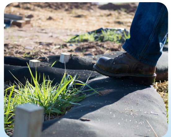
Compost-filled mesh socks help to control erosion and retain sediment in construction areas. These erosion controls trap sediment and pollutants, while allowing filtered water to pass through.
